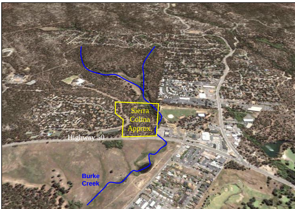
Figure 1. Approximate Alignment of Burke Creek Looking Upstream
